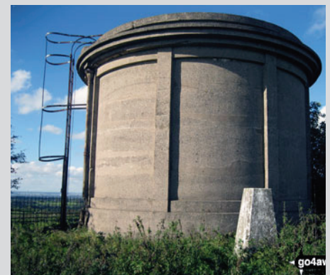
Trig point next to the water tower
