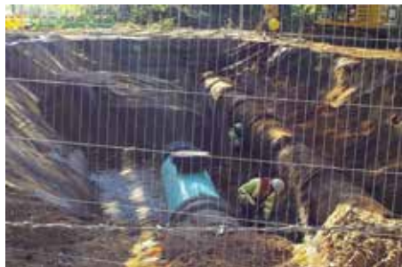
The new aqueduct pipes being installed
