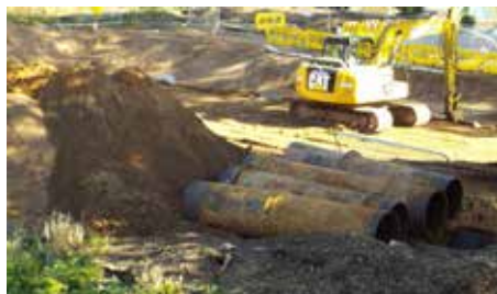
The old aqueduct pipes after removal
